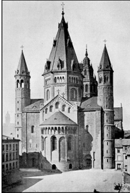
THE MAINZ CATHEDRAL in Germany typifies the Romanesque architecture with its heavy (thick) and relatively unadorned walls.
